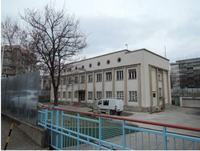
Ikarus Building in its current state
